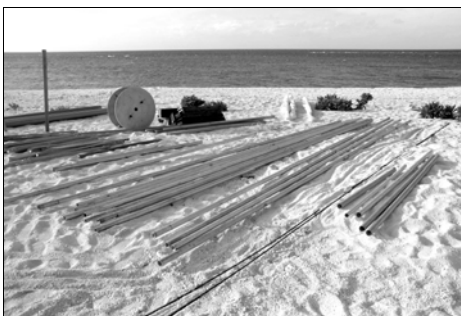
Masts for the beams - all at 40 feet
