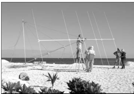
10m beam almost ready
